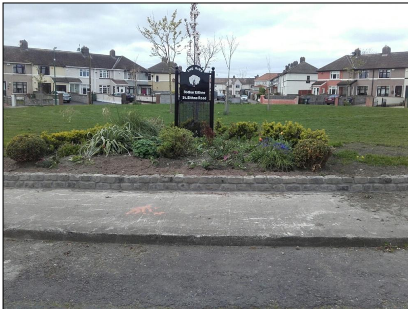
New kerbing installed around the green area on St. Eithne’s Road
